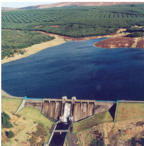
Altnaheglish Water Reservoir in Northern Ireland
